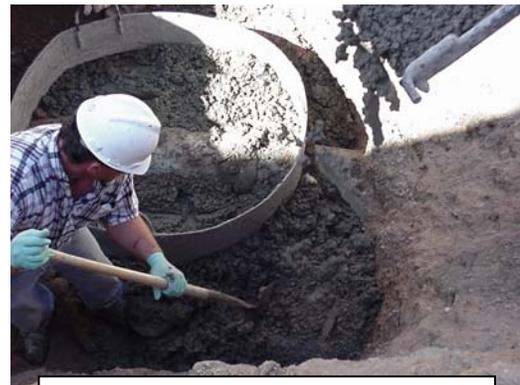
A workman places concrete around a manhole base
