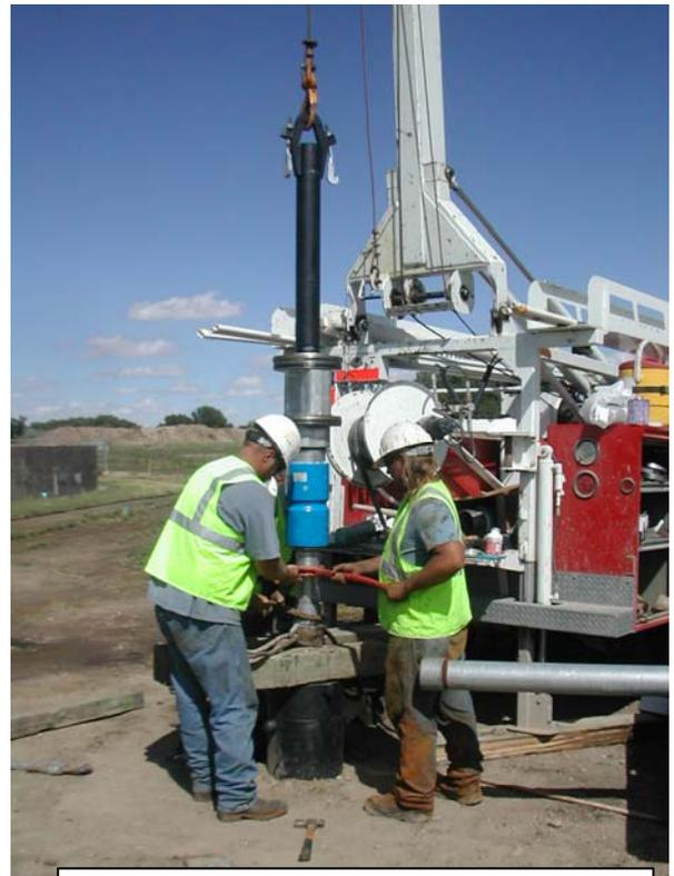
Drilling a well to lower the water table temporarily at the Water Reclamation Facility
