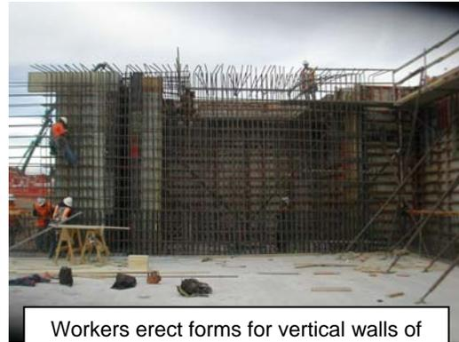
Workers erect forms for vertical walls of concrete tankage at the Water Reclamation Facility
