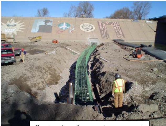
Construction of a concrete encasement for a 36-inch sanitary sewer main beneath the Arkansas River
