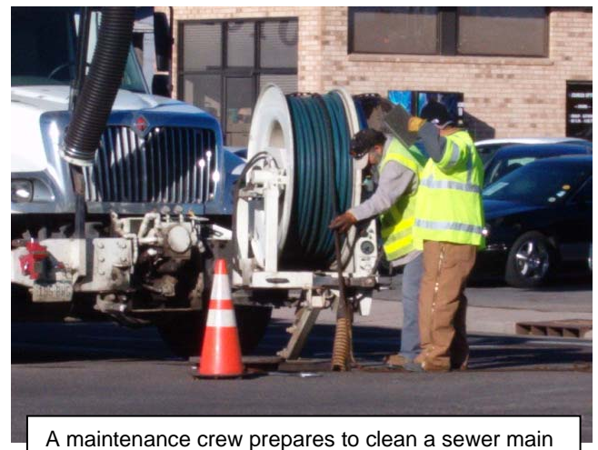
A maintenance crew prepares to clean a sewer main
