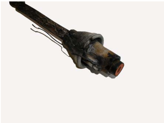
Photo ID: WW-03-2011Budget Capital Project: WRF Electrical Upgrade
