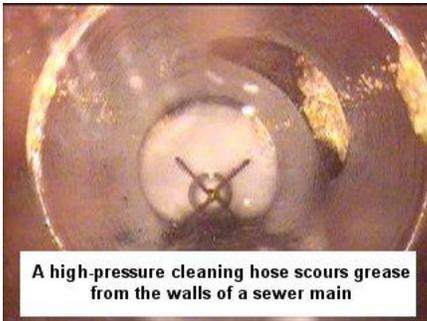
A high-pressure cleaning hose scours grease from the walls of a sewer main
