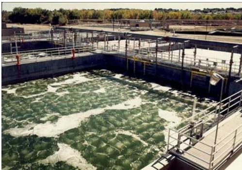
Early municipal wastewater treatment was done by primary treatment, which employs physical methods such as screens and gravitational settling in clarifiers to remove settleable and floatable solids from raw sewage. Secondary treatment, a biological process was added to remove a much larger amount of organic material. Each phase has added costs. As we learn more about the environmental impact of growing amounts of wastewater, chemicals used in urban
