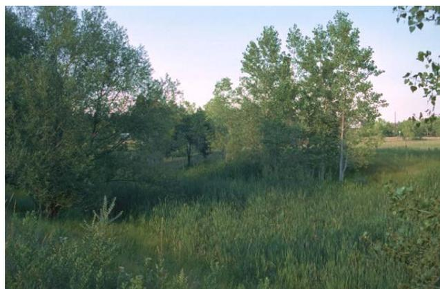
**Photograph 3-4.** An engineered wetland channel can serve as a filter for low flows and carry the major flood event without damage. Wetlands and vegetated overbank areas aid in providing transient storage that is beneficial for attenuating runoff.
