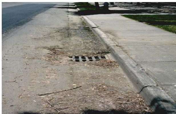
**Photograph 7-6.** Clogging is an important consideration when designing inlets.
