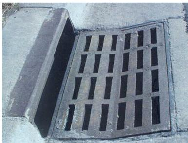
(a) CDOT Type 13 grated inlet in combination configuration
