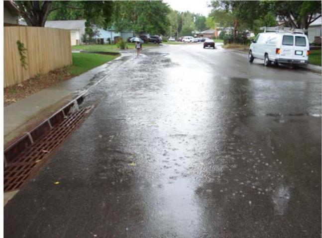
**Photograph 7-6.** Weir performance decay can be observed in this picture as flow appears to enter only the first two inlets while exceeding the height of the upstream curb.
