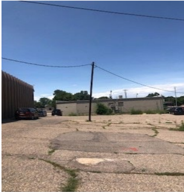
Tower site, view from Sumner looking northwest
