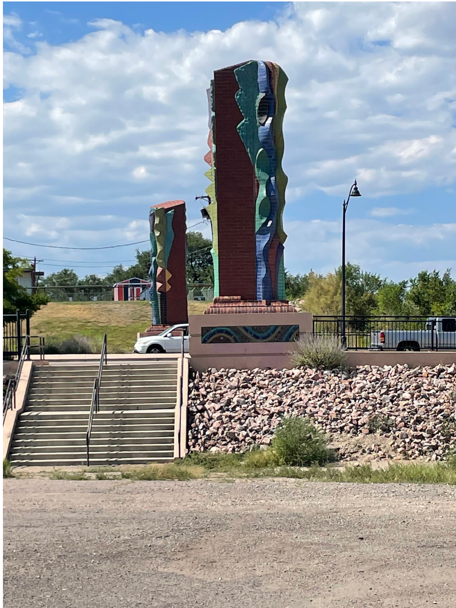
Brick and sculpted tile monument art installations located on the W. 4 th Street Bridge abutments
