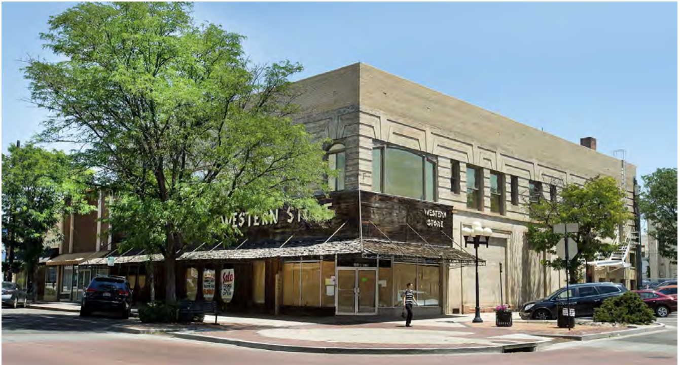
(E) SITE PHOTOGRAPH, 2017
