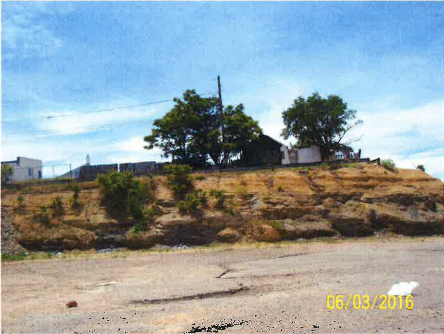
Alley from 302 E. City Center Drive
