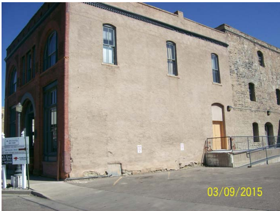
Photo #2. Overview of the side façade.
