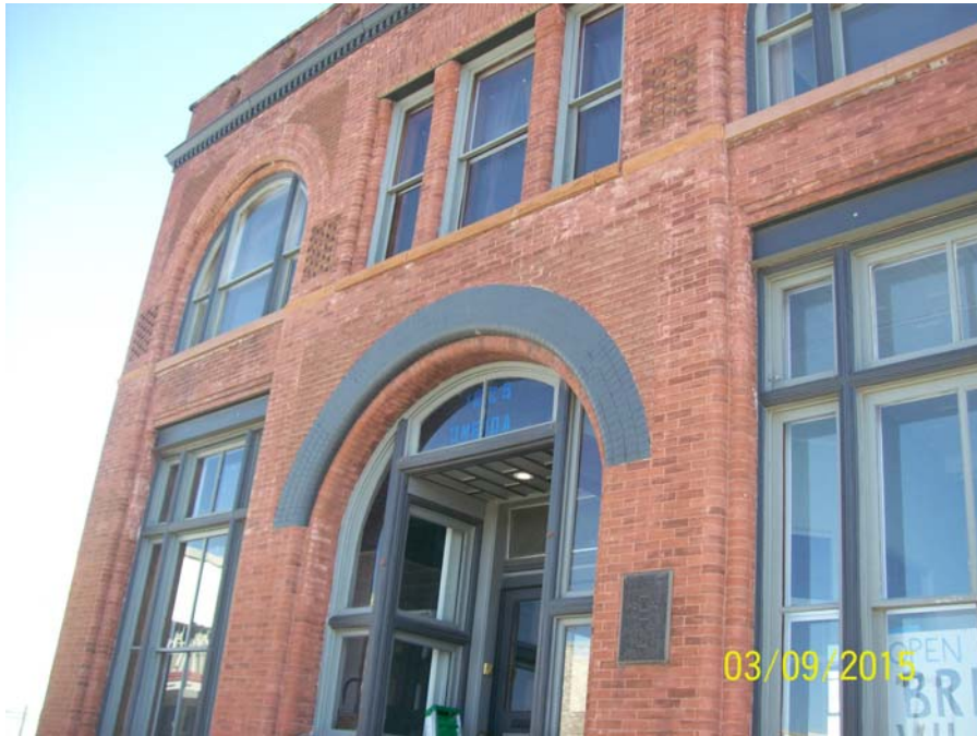
Photo #1. Overview of the Oneida St. façade.
